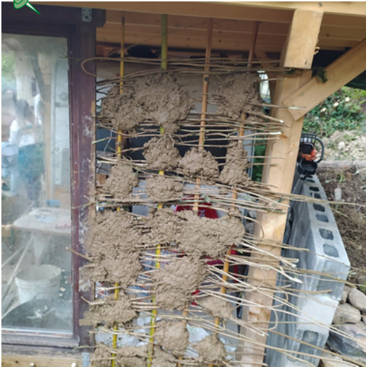
Building a cob wall
